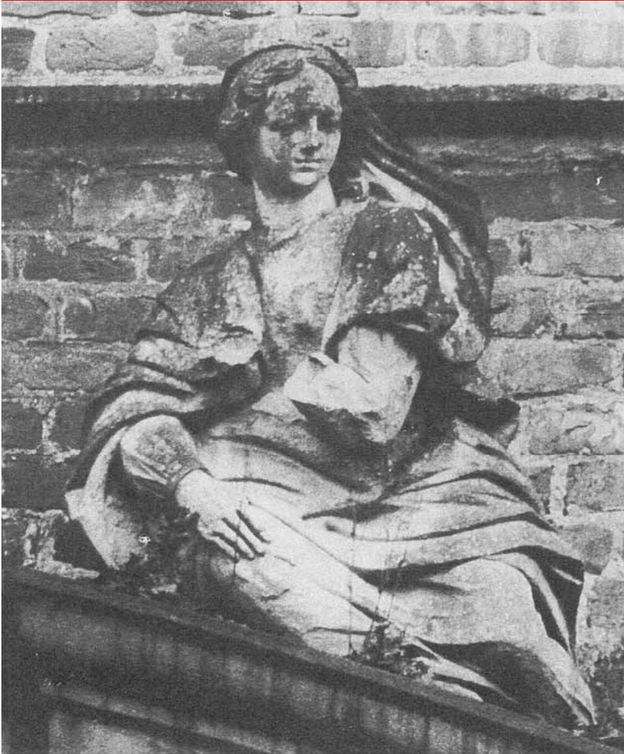
Figure 2.2.1 German ornamental figure made of sandstone. The figure, from 1702, is found at the Herten Castle in the outskirts of the Ruhr area. The picture on the left shows how the figure still looked in 1908. On the right one can see what had happened to the figure 60 years later (picture taken in 1969). It is a telling proof of how the stone has weathered under the damaging influence of serious air pollution (source: Westfälisches Amt für Denkmalpflege, Münster)
